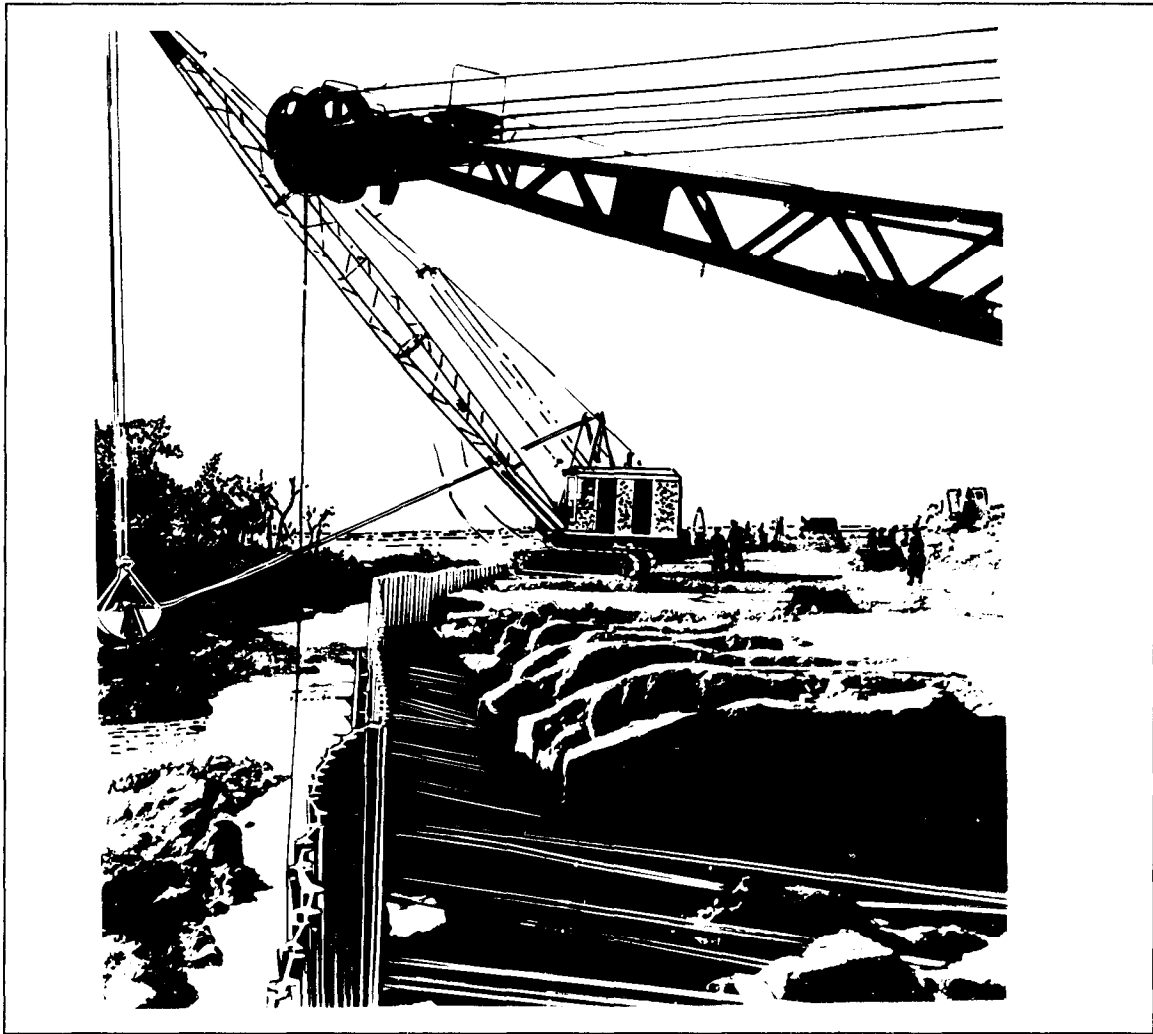
Figure 7-1. Bulkhead Using Steel Sheet Piles and Tie-Rods
